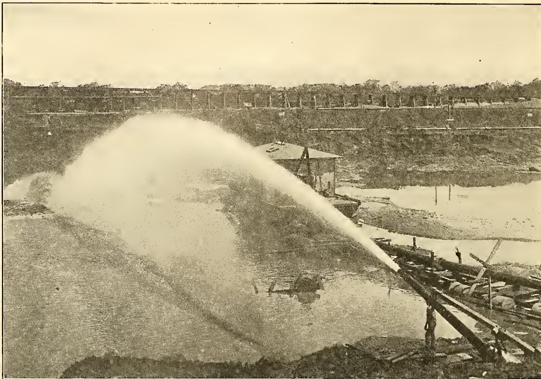
EXCAVATING WITH A MONITOR AS CALIFORNIANS DIG GOLD
